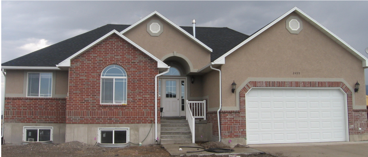
Photo shows client changes
